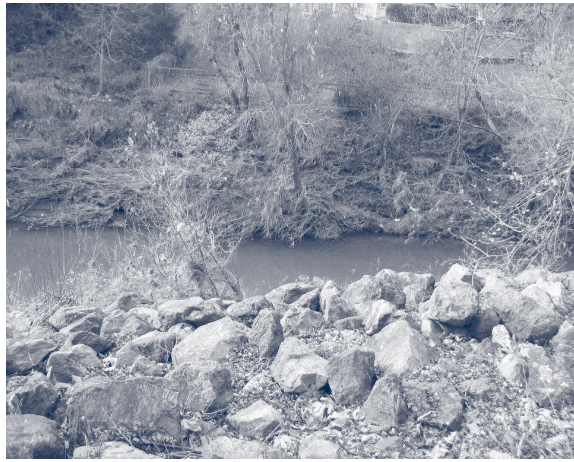
This is an example of a creek with incised banks.
