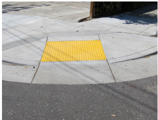
Figure 4-3: Curb ramp with detectable warning strip
