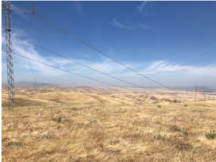
Location AUC-01, looking north.
