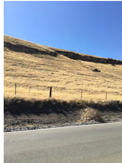
Location AUC-08, looking west.
