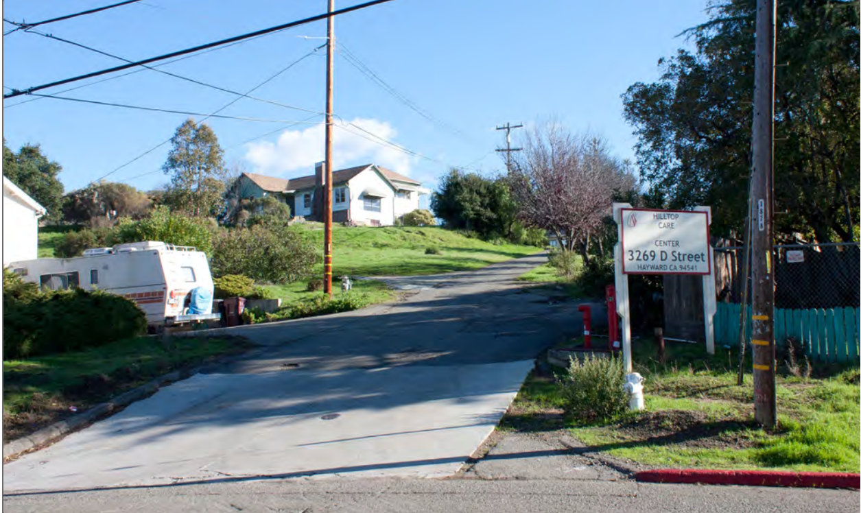
Existing view from D Street near Carlson Court looking southeast
